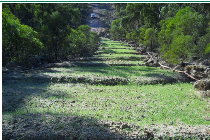
Corridor re-vegetated with grasses and stabilised with erosion-prevention structures, which will in time be re-colonised with suitable tree species (images Beneterra, 2017)
