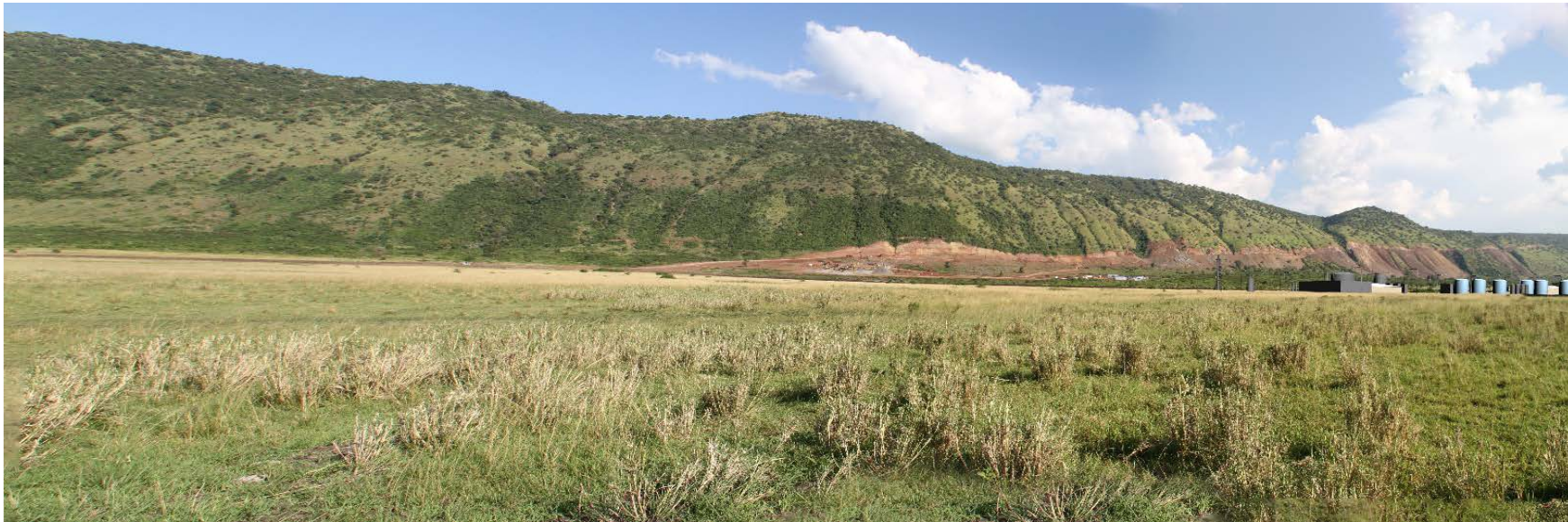
Figure 20: Daytime view of the CPF site from the northwest, after construction of the project infrastructure
