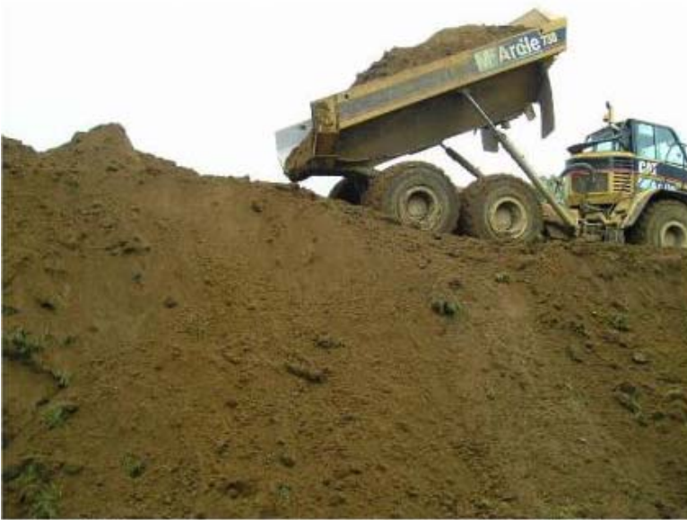
Figure 24: Stockpiling topsoil.
