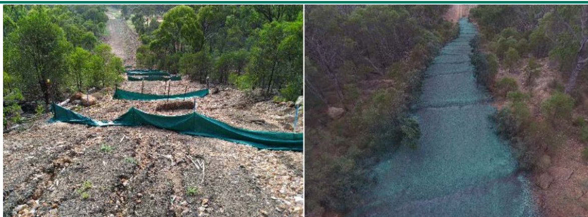
Initial backfilled pipeline corridor along a steep embankment protected against erosion with mulch and sediment netting (left) and subsequently soil binding polymers (right)
