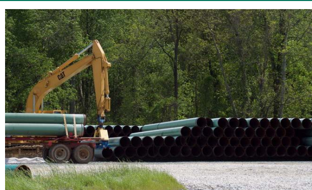
Temporary pipeline and material laydown area
