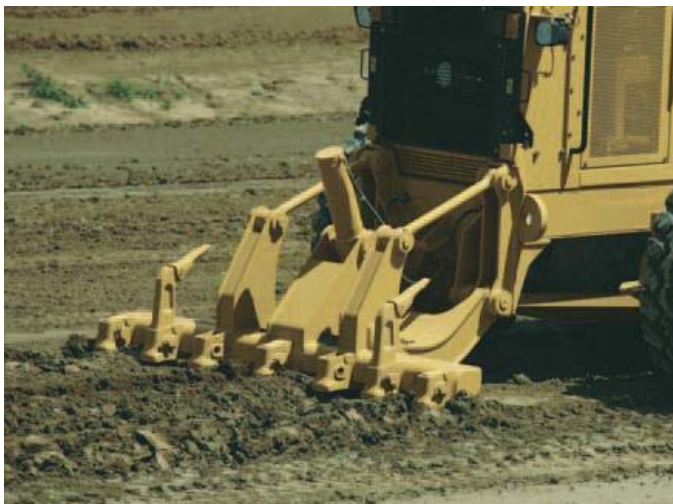
Figure 26: Grader ripping compacted soil.
