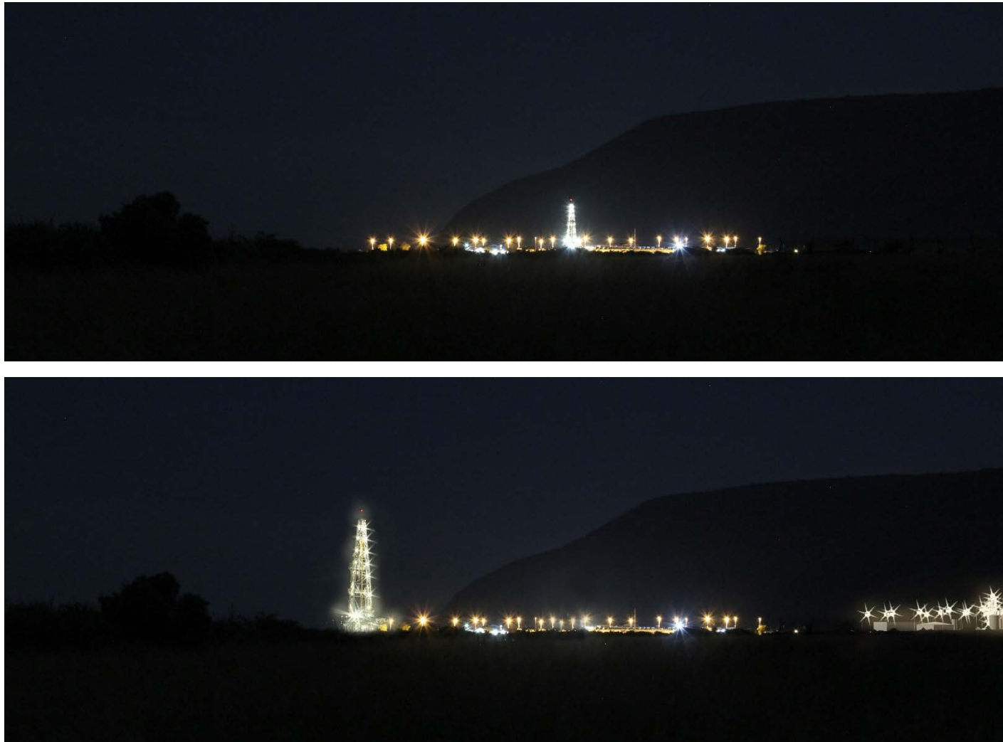
Figure 22: Night-time view of the permanent camp, CPF site and well pads 1 and 2 positions, before (top) and after (bottom) construction of the project infrastructure
