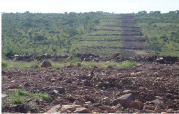
Reinstated surface with drainage berms
