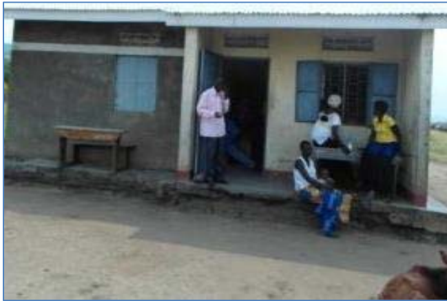
Photograph 6-27: Buhuka Health Centre III
