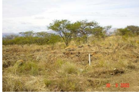
Reinstated surface with pipeline centreline marker
