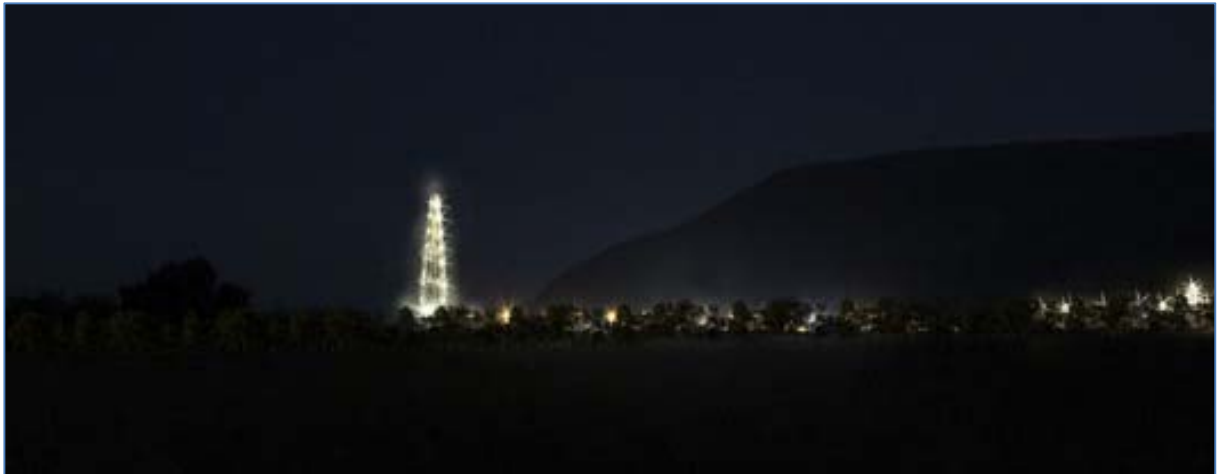
Figure 8-12: Night time view of Drilling Rig 1, the permanent camp and the production facility after screening
