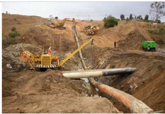
River crossing (note flume pipes)
