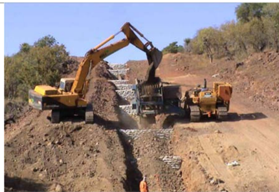
Trench breakers on steep slopes
