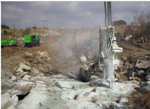
Blasting in rocky areas
