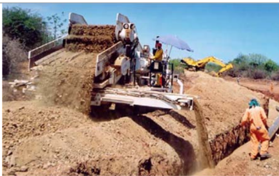
Screening plant backfilling the trench
