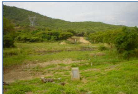
Photograph 2-3: CP Post along a pipeline route
