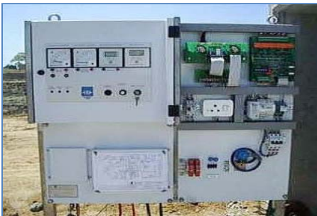
Photograph 2-2: CP instrumentation. The instruments provide information to maintenance teams which demonstrate that the cathodic protection is working properly.
