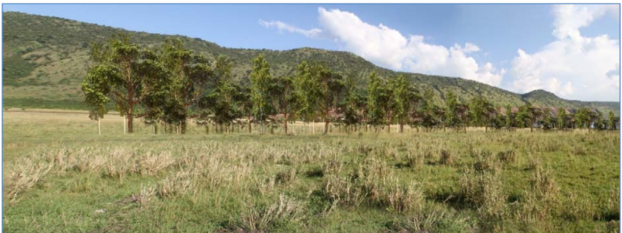
Figure 8-13: Daytime view of a tree screen viewed from the north-west back towards the CPF (screened CPF oil tanks in the far right)
