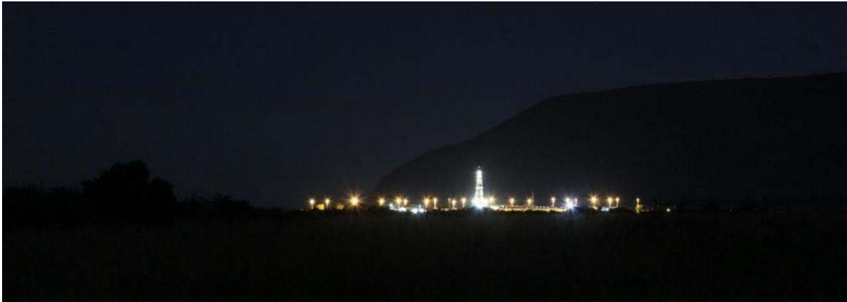
Figure 7-10: View of night lighting at the CPF construction site and a lit drilling rig on well pad 1
