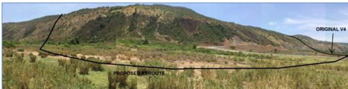
Figure 16-2: Kingfisher feeder pipeline re-route near the CPF
