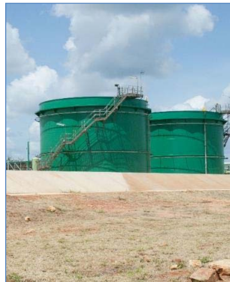
Photograph 2-4: Typical stabilised oil floating roof storage tanks
