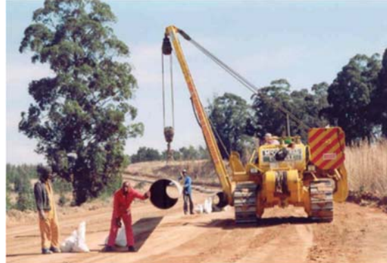
Pipe string along the RoW
