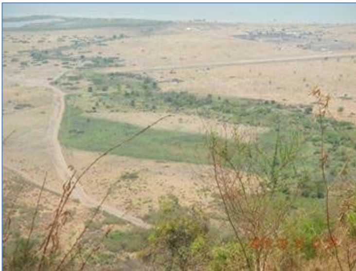
Photograph 8-5: Impact of a poorly designed road on the Kamansinig Wetland
