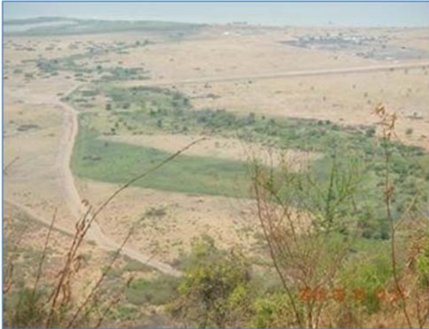
Photograph 6-20: Indication of poor road design and insufficient culverts negatively affects hydrological flows and resultant deterioration in wetland function
