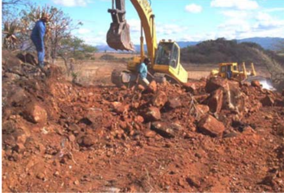
Clearing and grubbing
