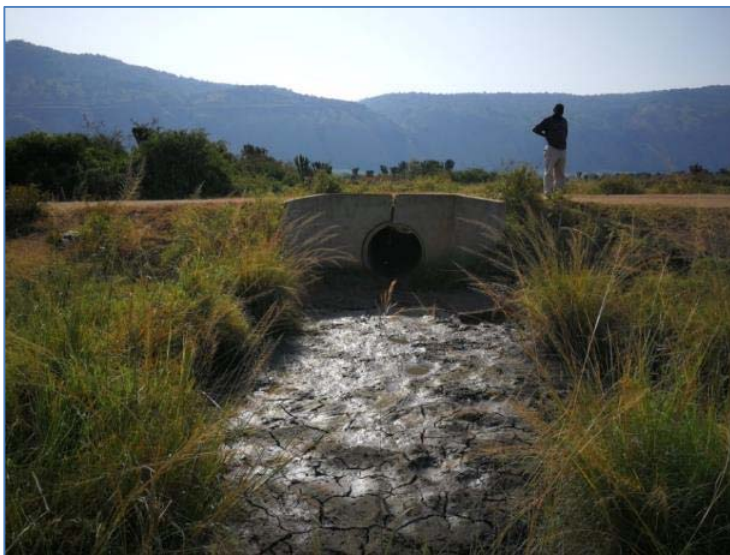
Photograph 8-4: Road culvert across the subsidiary channel of the Kamansing River
