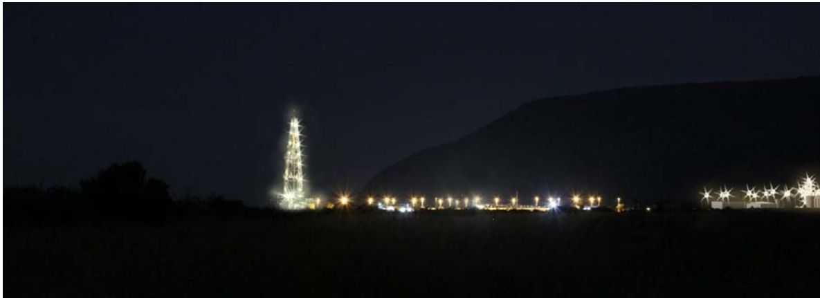
Figure 8-10: View of night lighting at the CPF production facility and a lit drilling rig on well pad 1
