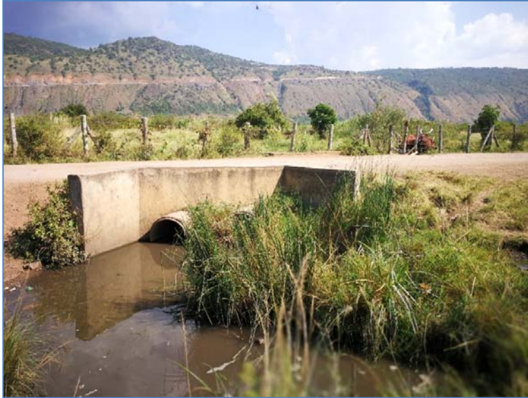
Photograph 8-3: Road culvert across the main channel of the Kamansing River
