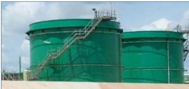
*Photograph 2-2: Oil will be stored in 10,000 m<sup>3</sup> tanks with floating roofs. Temperature in the tanks will be maintained at 68°C.*
