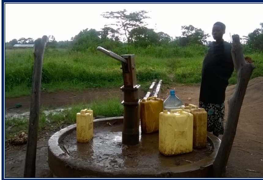
Figure 28: Community handpump well in Kyarujumba
