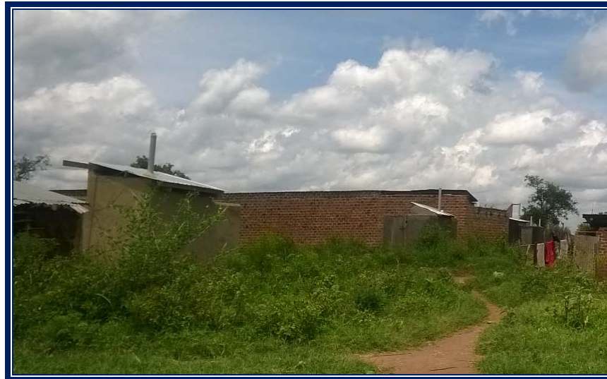
Figure 29: Vented improved pit latrines in Kyarushesha
