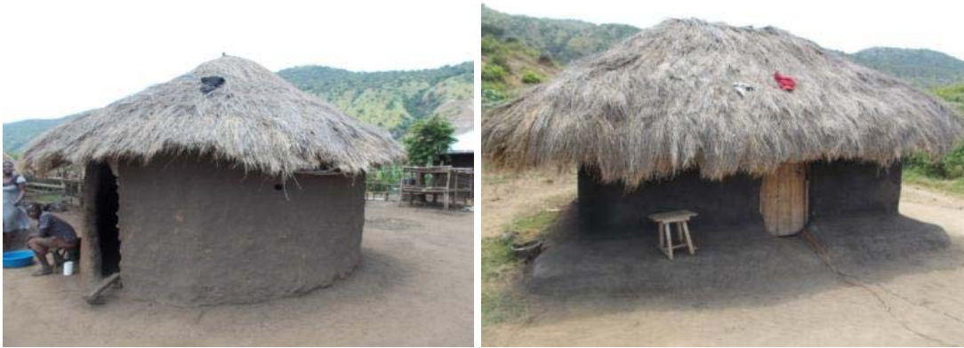
Photograph 11: Semi permanent structures used as a kitchen (left) and for accommodation (right)
