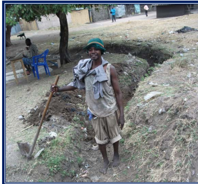
Figure 21: Clearing drainage ditches
