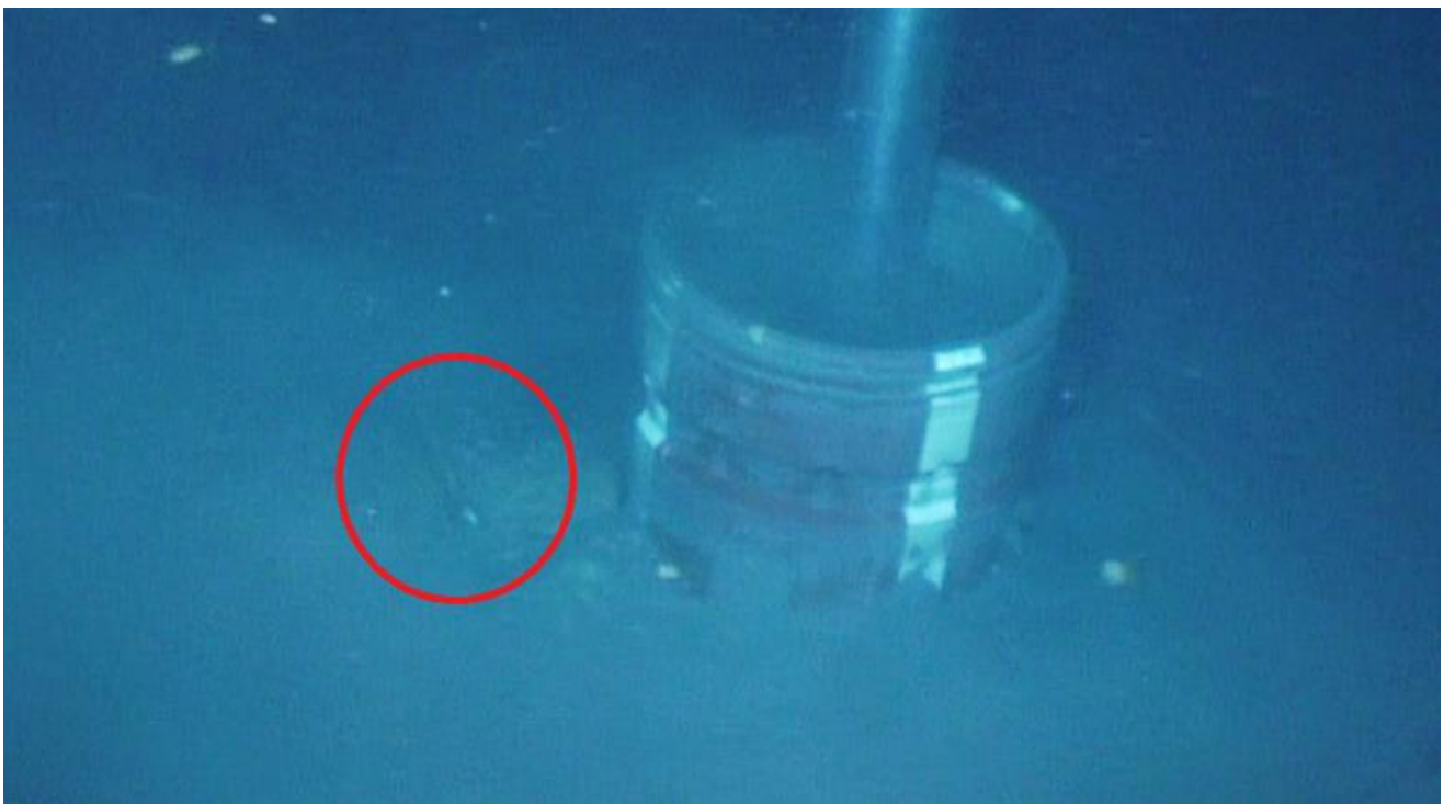
Figure 3-5 Image showing the 1.5 m accumulation of drill cuttings around the wellhead. The ball valve (circled) is flush with the cuttings level and is located 1.5 m above the seafloor.
