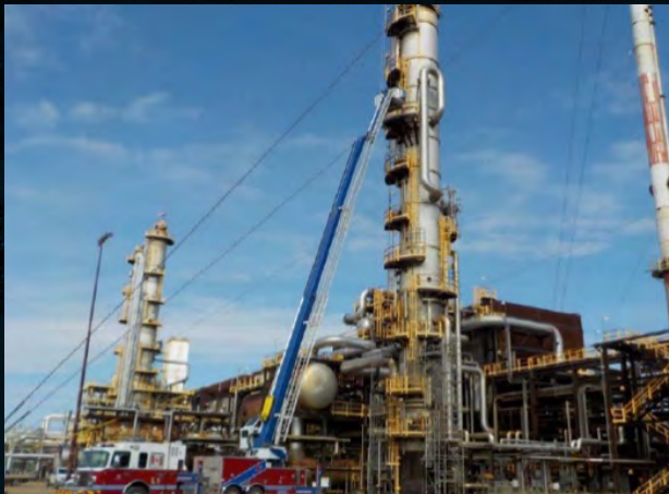
The intricacies of our full-scale drills and the equipment and machinery used
