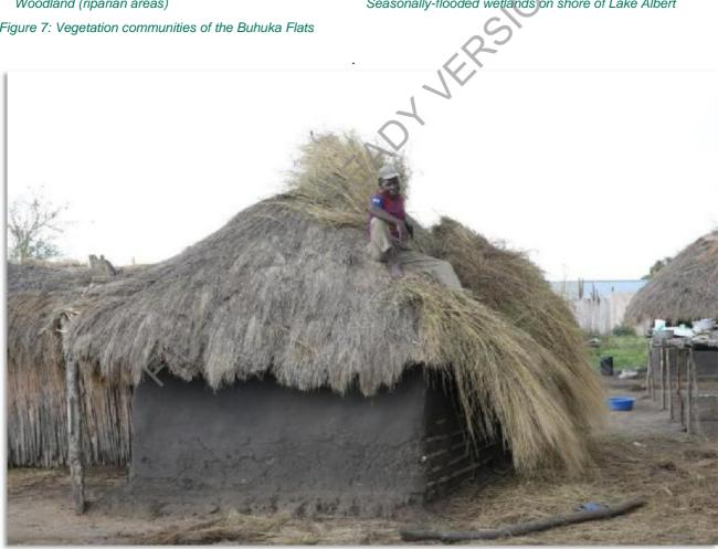
Figure 8: Traditionally built house in process of being thatched
