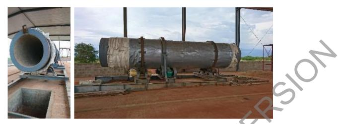
Figure 13: Dual-chamber Rotary Kiln under Construction at Luwero's Facility
