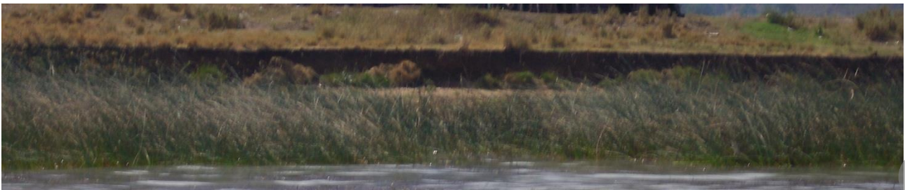
Figure 12: Wave erosion occurring on the shoreline of the Flats
