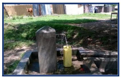
Figure 26: Functional gravity fed water tap in Nsonga
