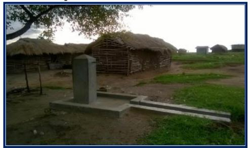
Figure 25: Non functional tap from gravity fed water scheme in Kacunde
