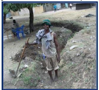
Figure 21: Clearing drainage ditches
