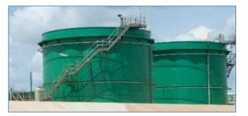
Photograph 2-2: Oil will be stored in 10,000  $m^3$  tanks with floating roofs. Temperature in the tanks will be maintained at 68°C.
