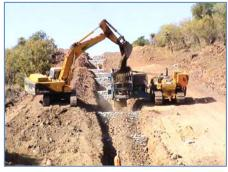
Trench breakers on steep slopes
