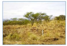
Reinstated surface with pipeline centreline marker
