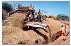
Screening plant backfilling the trench
