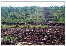
Reinstated surface with drainage berms
